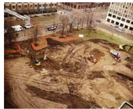
LEVITT PAVILION DAYTON CONSTRUCTION SITE
