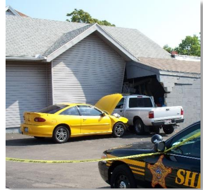
Unexpected damage can cause serious disruptions
